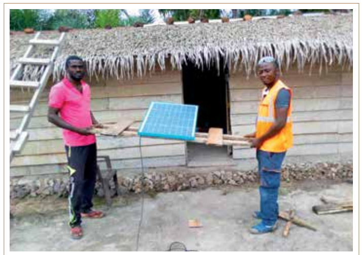
Installation of BBOXX Kits in Malibé.
